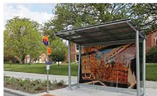
Improved the customer experience and featured public art through the installation of new art bus shelters
